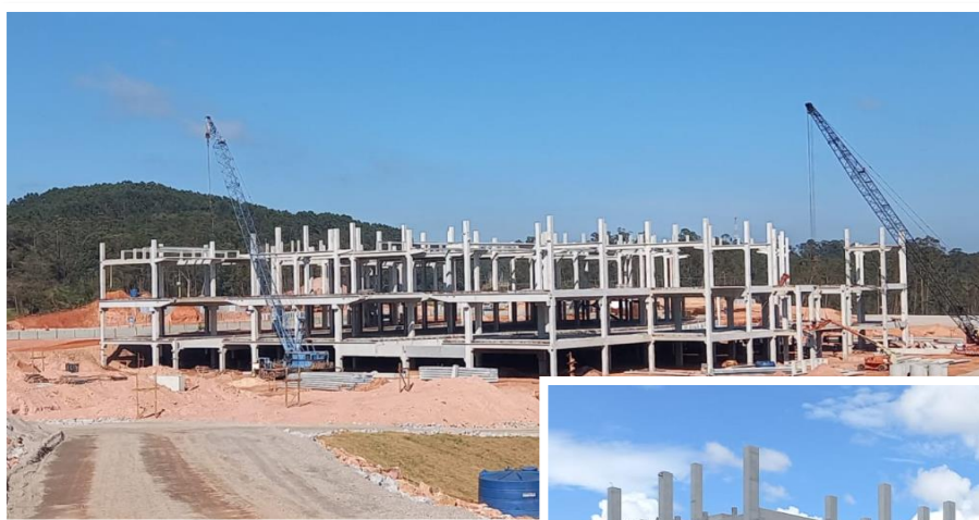
CFO expansion works
